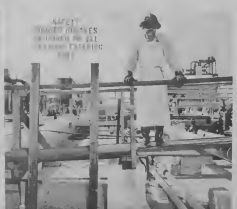
CLEANOUTMEN USE rubber boots and gloves, rubber type goggles and apron against corrosive chemicals. TRAHADOR DI Cleanout ta usa botas y handschoen di rubber, bril y lantera contra quimico corrosivo.
